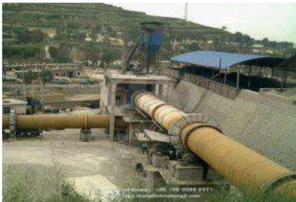
Figure 1. Gypsum production plant rotary kiln view (enterprise capacity 50-400 tons per day)
